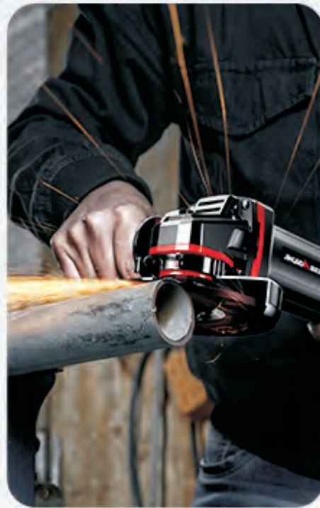
STEEL PIPE GRINDING
