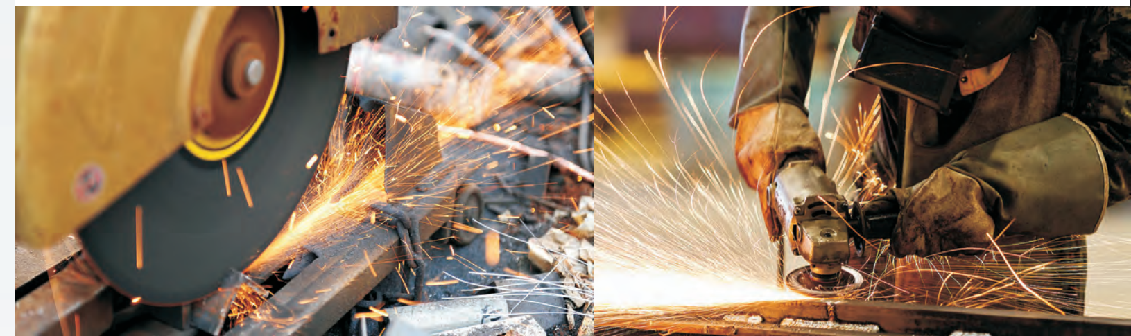
CUTTING ANGLE IRON
